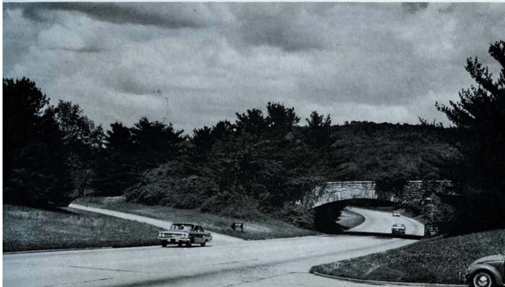
A typical parkway of the 1920s in Westchester County, N.Y.
