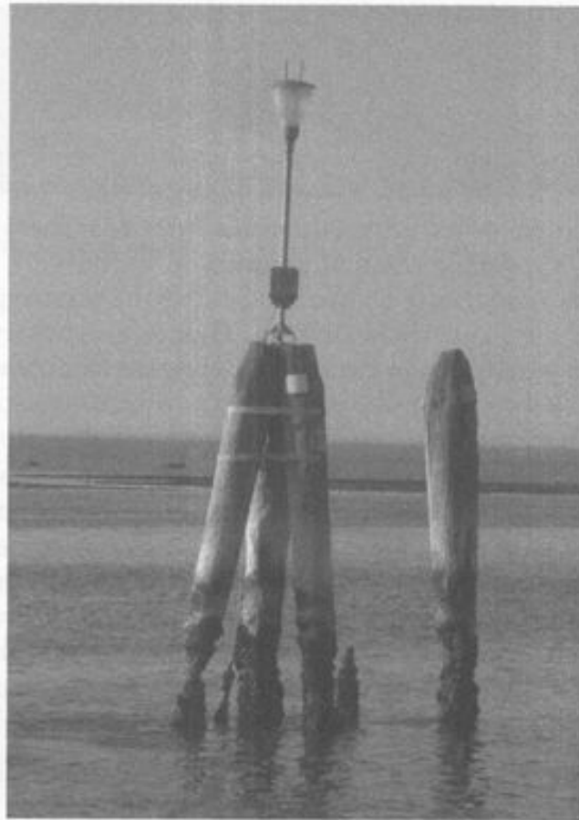
Figure 30.3 The sculptural shapes of rotting bricole are well visible at low tide.
