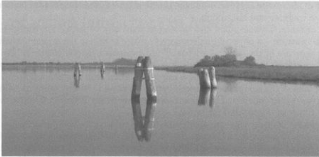
Figure 30.4 Wooden and concrete bricole .
